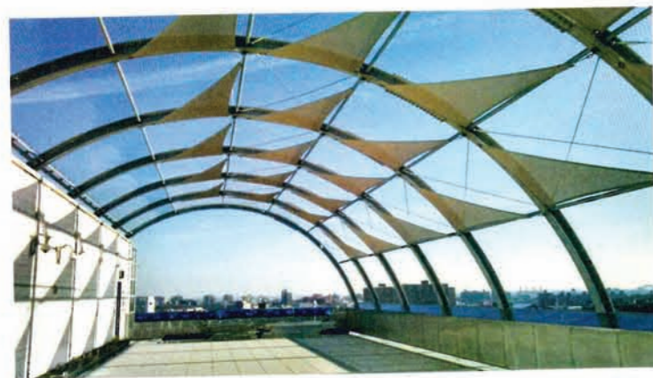
For a school for gifted children's 15th-floor rooftop playground in Manhattan, N.Y., Capitol Awning Co. designed and installed 24 triangular shade sails manufactured with mesh PTFE. The non-stick surface resists pollution, an important component for the New York City installation. Photo: Capitol Awning Co.
