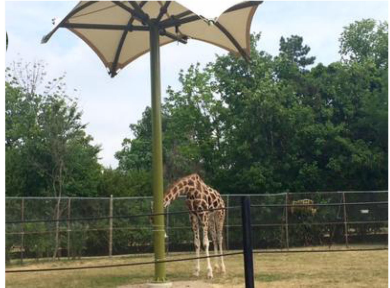
Brand new giant umbrella-like structure in the Giraffe exhibit gives much needed shade for giraffes.
